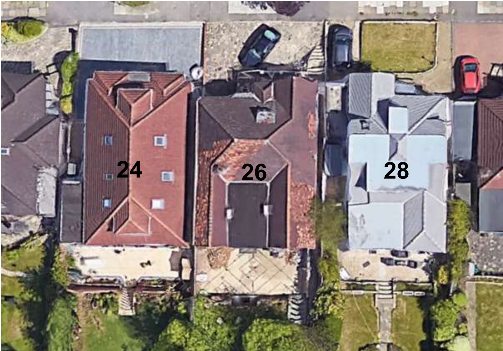
AERIEL VIEW Showing major roof alterations of neighbouring dwellings 22, 26 and 28 Hillside Road.
