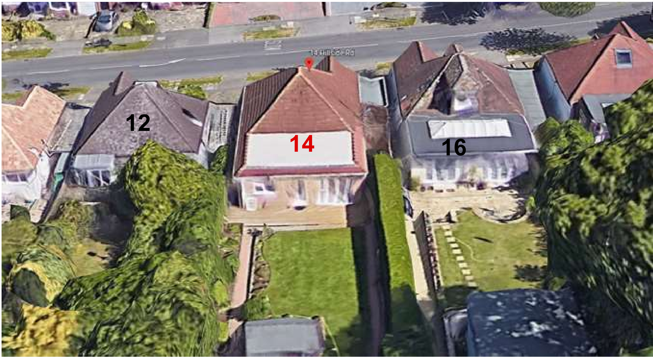
REAR VIEW Showing 14 Hillside Rd with neighbouring properties
