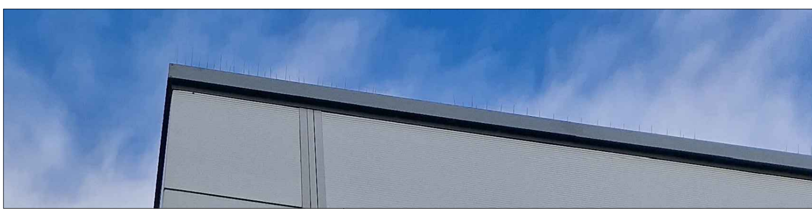
Powder coated aluminum parapet trims - Colour - RAL: 7012
