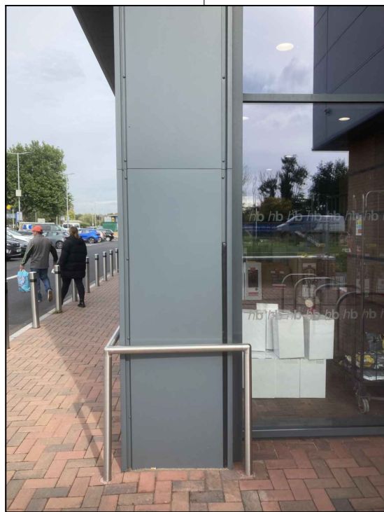
GREY COLUMN ENCASEMENT
