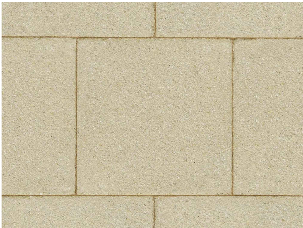
IMAGE SHOWING MARSHALLS SAXON 450mm X 450mm PAVING FLAGS INSTALLED TO ENTRANCE AREA
