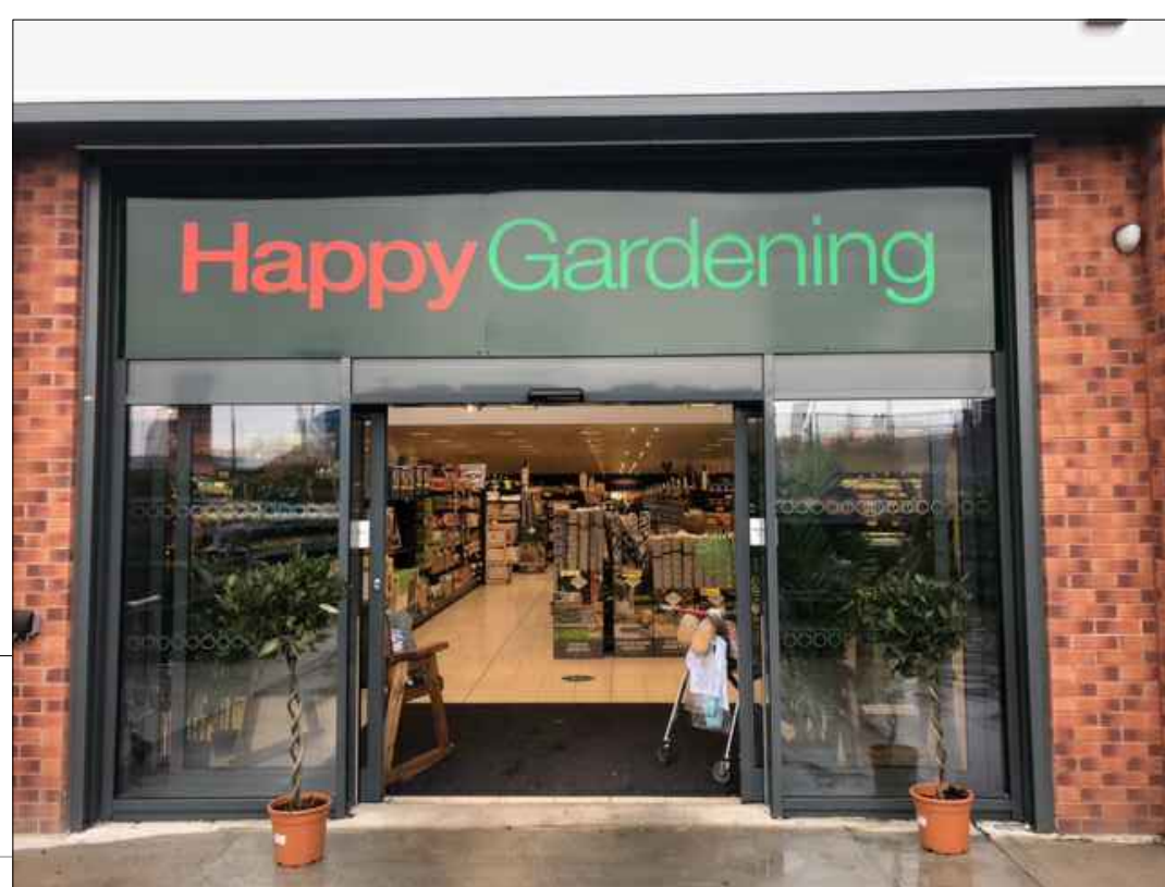
Powder coated aluminum frame Garden center bi parting glazed doors. Colour: Grey - RAL: 7011
