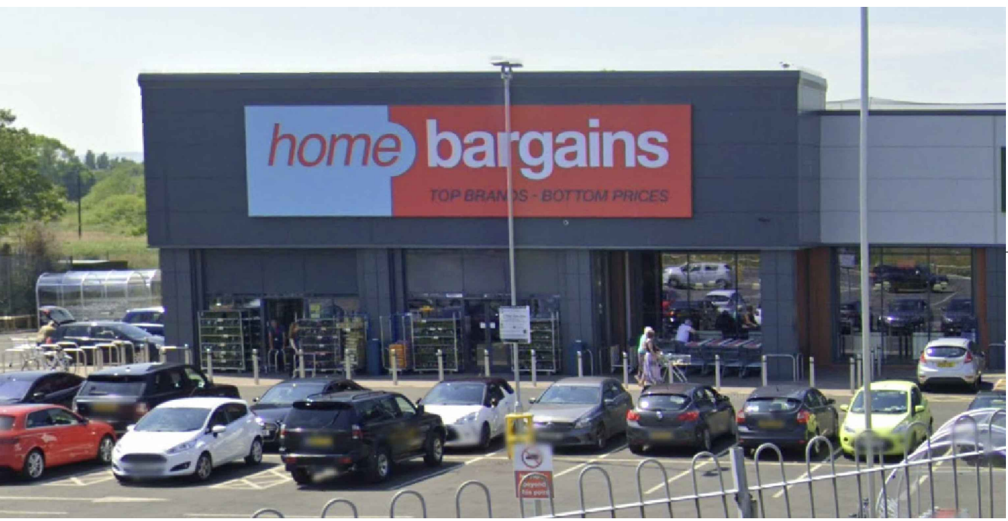
SIMILAR HOME BARGAINS ENTRANCE FEATURE
