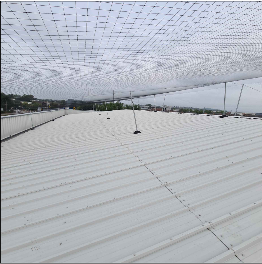
KINGSPAN KS100RW TRAPEZOIDAL ROOF SHEETING AND WALL PANELS TO REAR OF PARAPETS, WITH MATCHING ASSOCIATED TRIMS AND FLASHINGS, COLOUR RAL 080 70 05 / BS 10A05 (GOOSEWING GREY)
