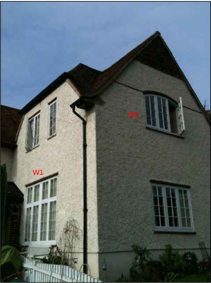
CORNER PHOTO OF BUILDING SHOWING WINDOWS TO BE UPGRADED.
