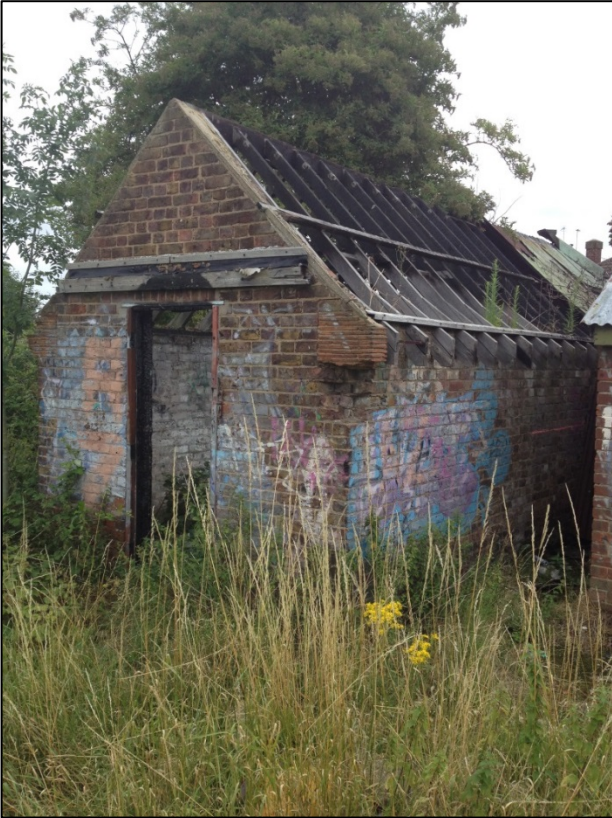
Plate 5: Building 2 south-west aspect (View: north-east)
