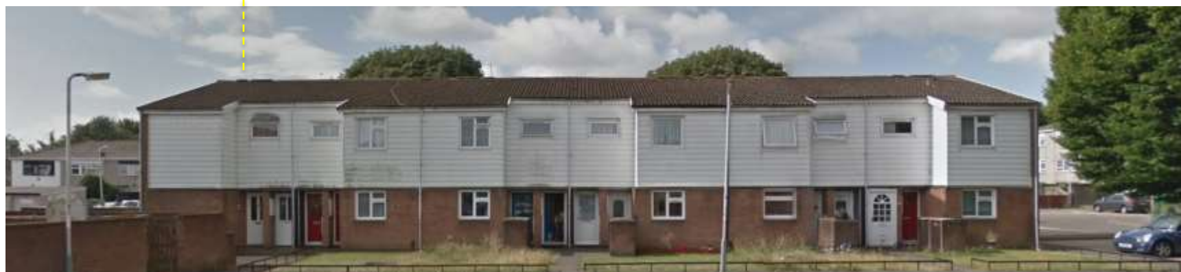
Typical 2 storey terrace block
