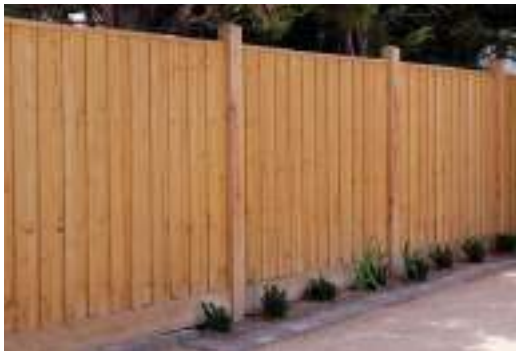
F1 – TYPE ONE 1800MM HIGH TIMBER BOARDED FENCE
