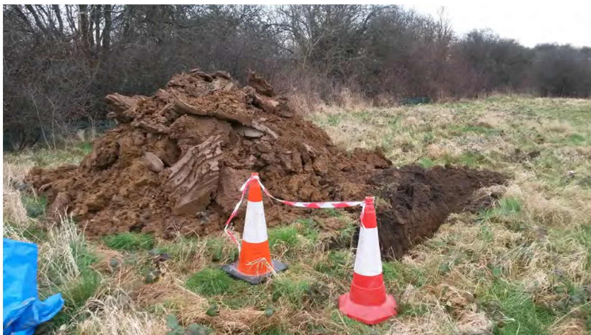
Photograph 11: Location of TP02 and encountered materials.
