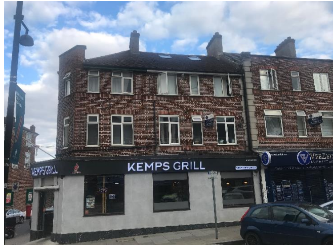
Figure 1: Front view of Kemps Grill, 31 Joel Street, Northwood Hill, HA6 1NU.
