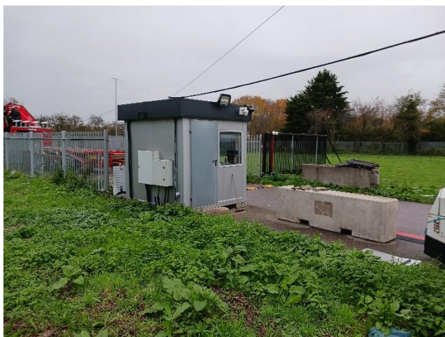
Photograph 6 View Building B1, facing north-west.
