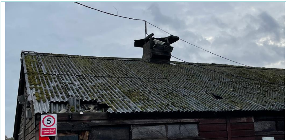
Image 12 Fibre cement Roof Covering
