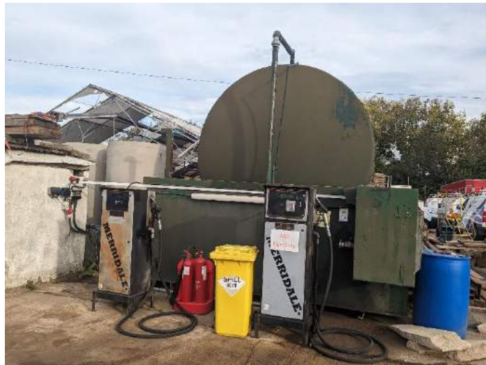
Photograph 8: Bunded 58000l Diesel tank with pumps. View looking north.
