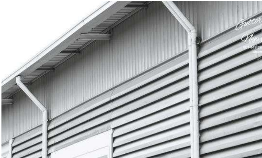
Figure 6:- Typical detail of extruded aluminium gutter system
