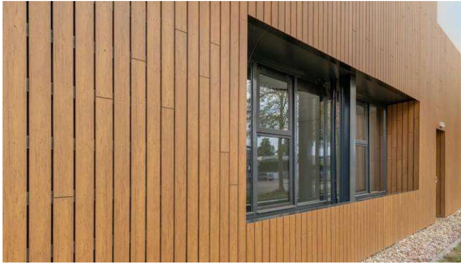
Figure 3:- typical image of Rockwool 'Rockpanel' cladding system
