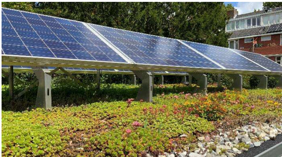
Figure 4:- typical image of green roof system, alongside solar panels
