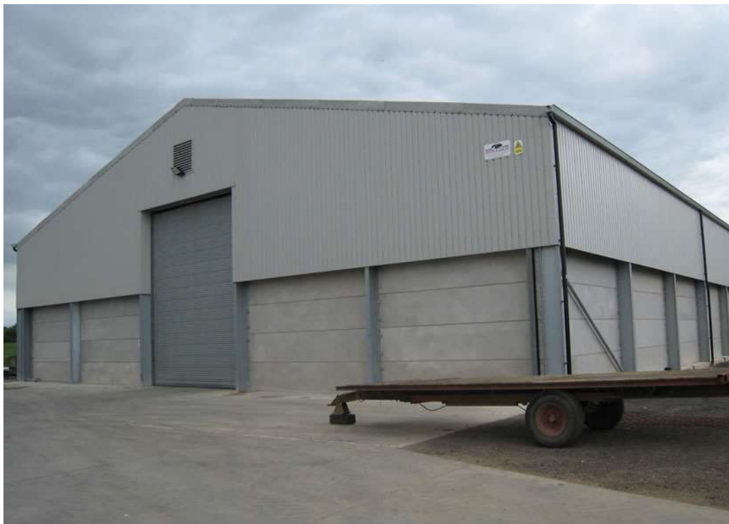
Figure 7:- Typical image of concrete wall panels with metal cladding above
