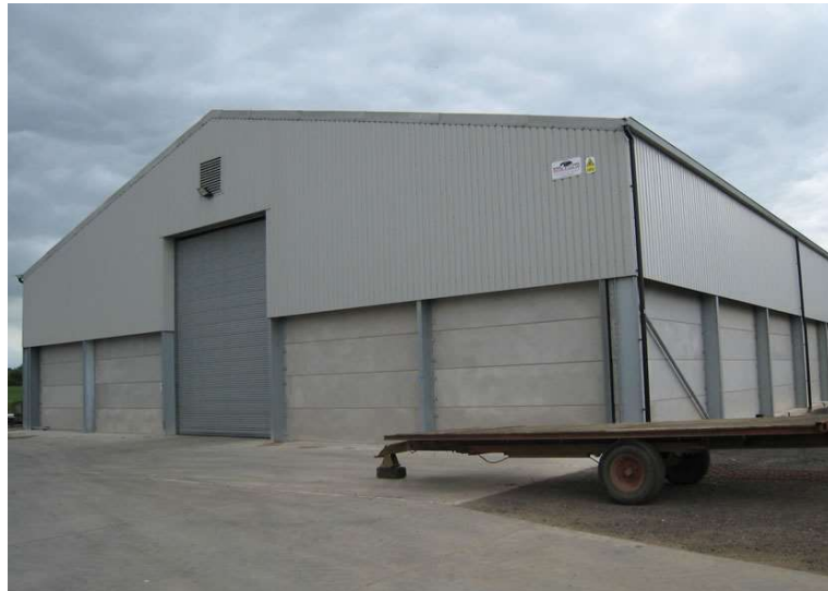
Figure 10:- Typical image of concrete wall panels and metal cladding above, proposed for service building
