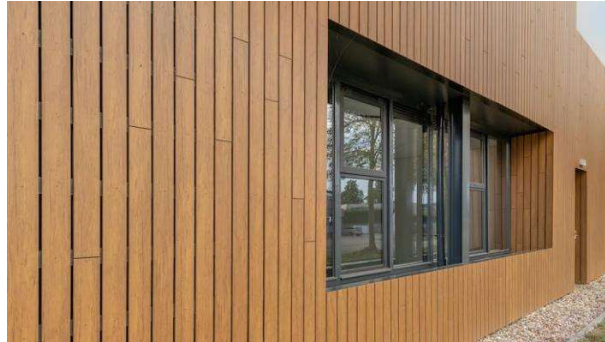
Figure 6:- typical image of Rockwool 'Rockpanel' cladding system, used on office building
