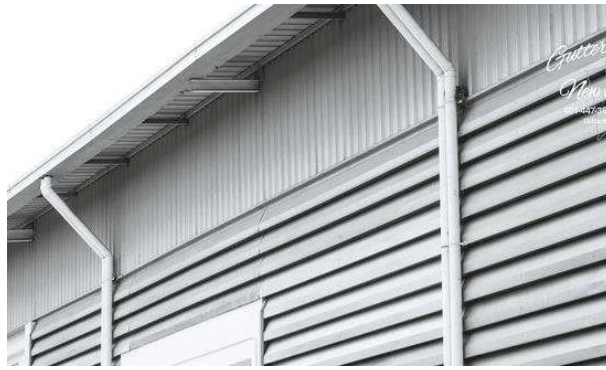
Figure 9:- Typical detail of extruded aluminium gutter system for both service and office building
