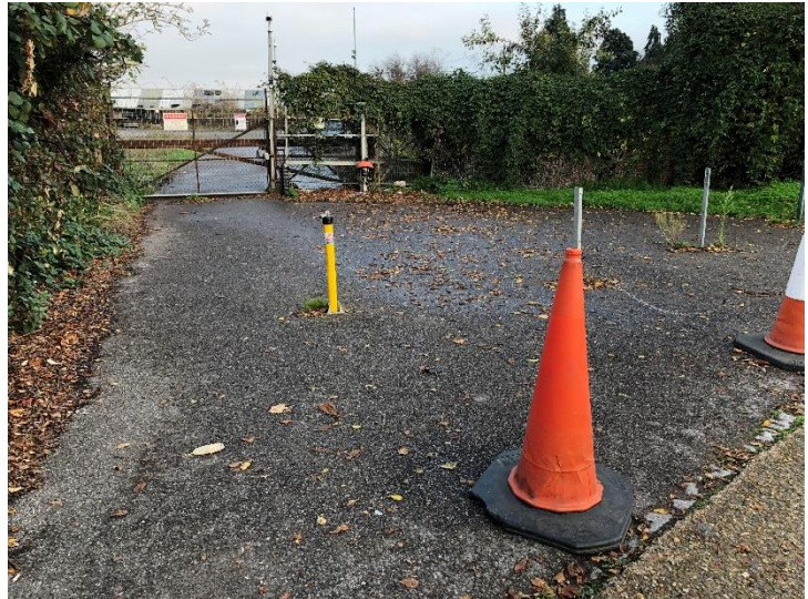
Photograph 2: Existing Access Arrangements
