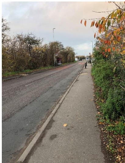
Photograph 5: Pedestrian footways north of the site access.
