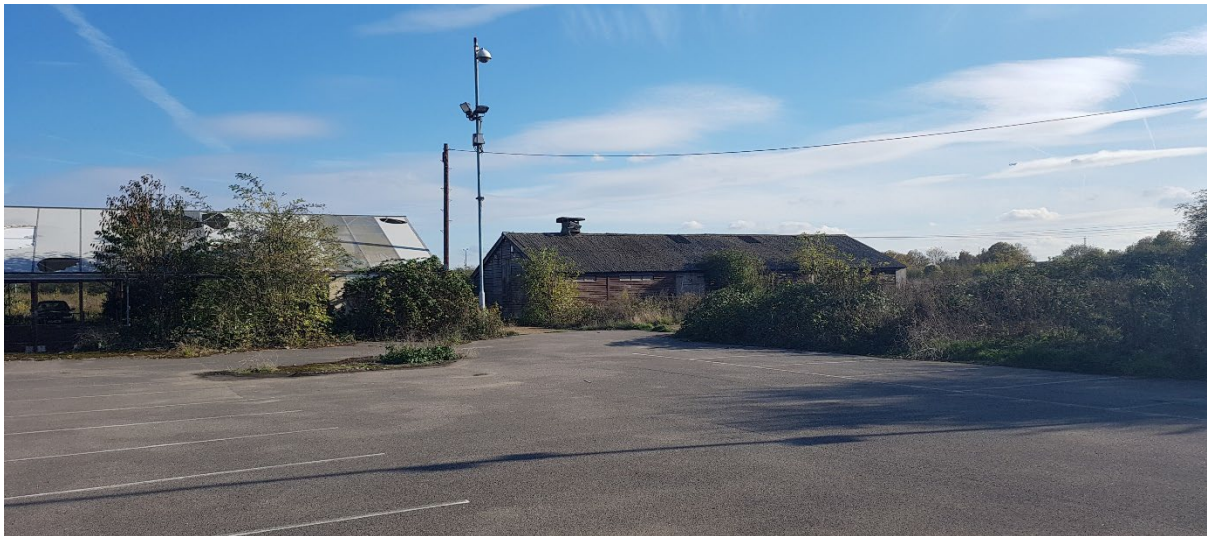
View of front (western side) of outbuilding from car park
