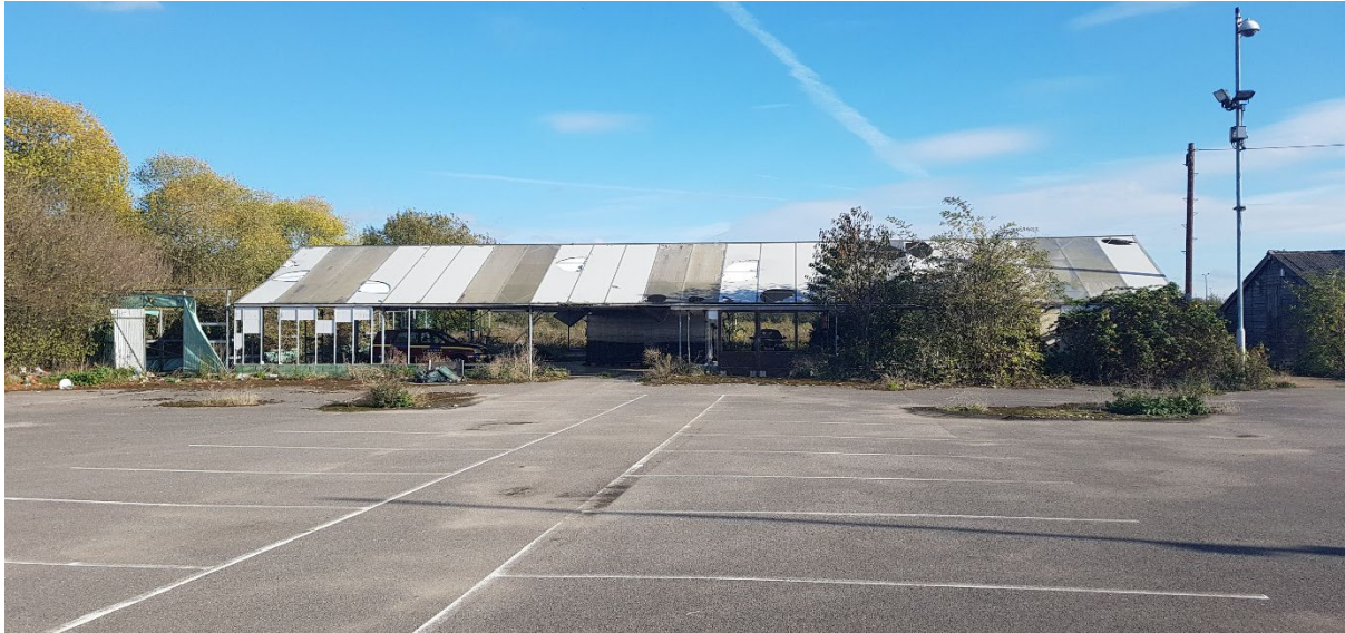
View of front (western side) of main building from car park
