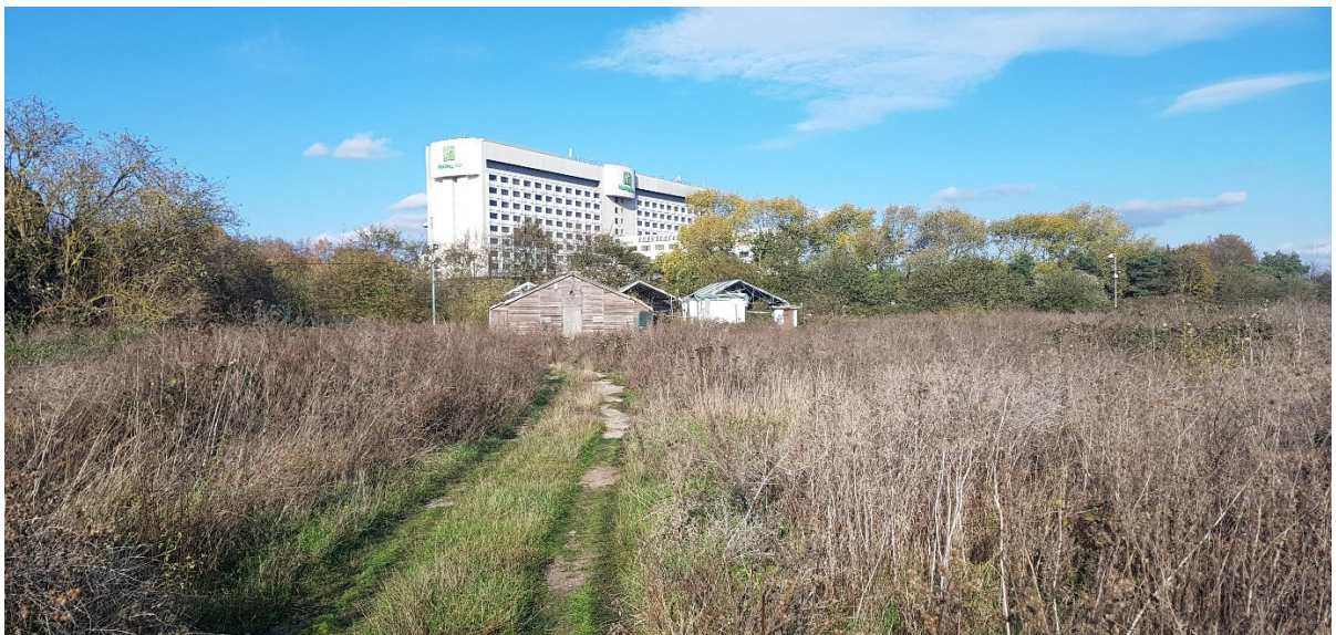
Southern view of existing buildings looking towards the north
