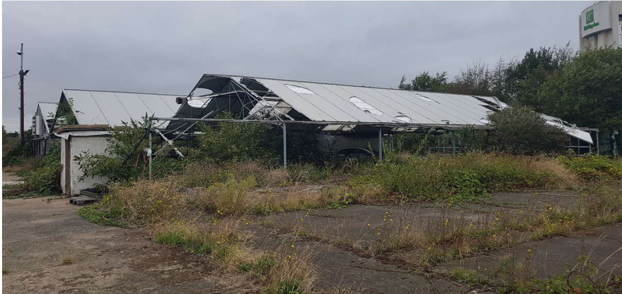
Close up view of eastern side of main building
