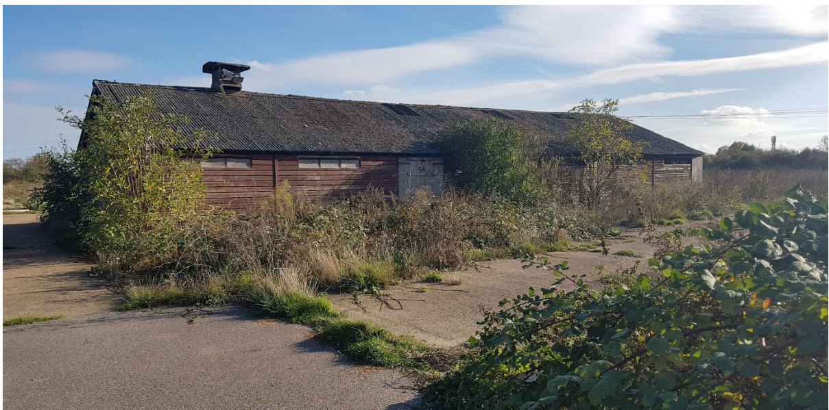
Close up view of western side of outbuilding
