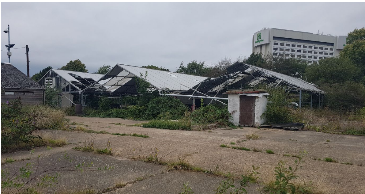
Close up view of eastern side of main building
