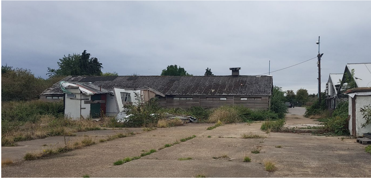
Close up view of eastern side of outbuilding
