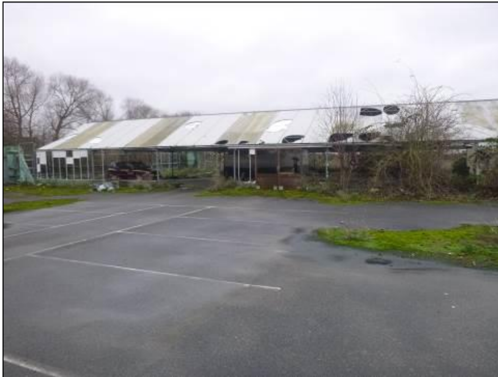
Photograph 1 Showing the derelict greenhouse on-site
