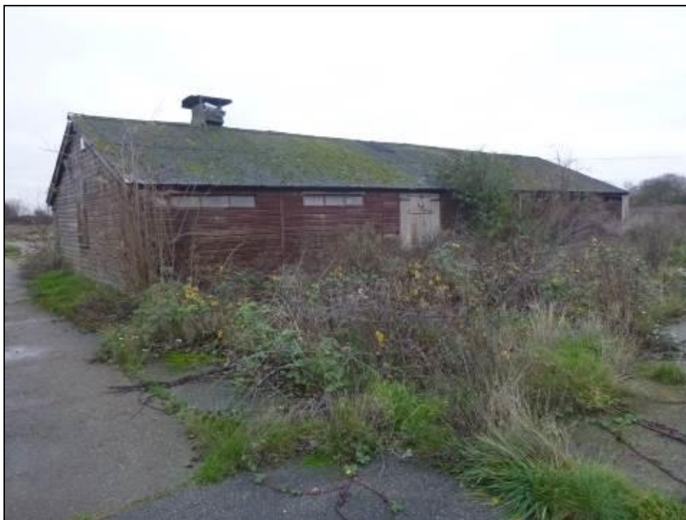
Photograph 2 Showing the timber outbuilding on-site
