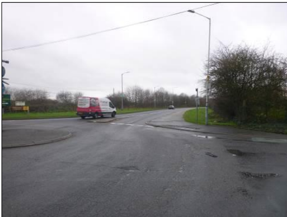
Photograph 8 Looking southwest along Holloway Lane
