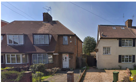
Typical properties in Harvey Road.
