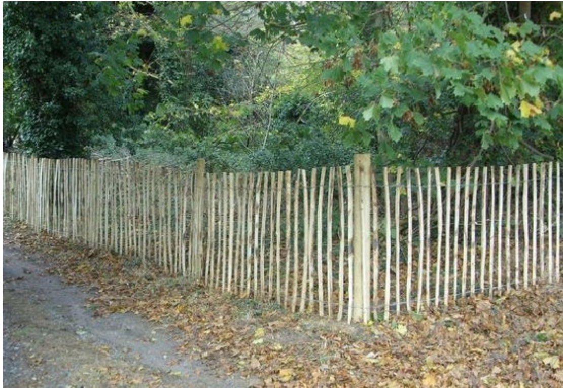
Fig. 1 Protective chestnut pale fencing supported by sturdy upright posts
