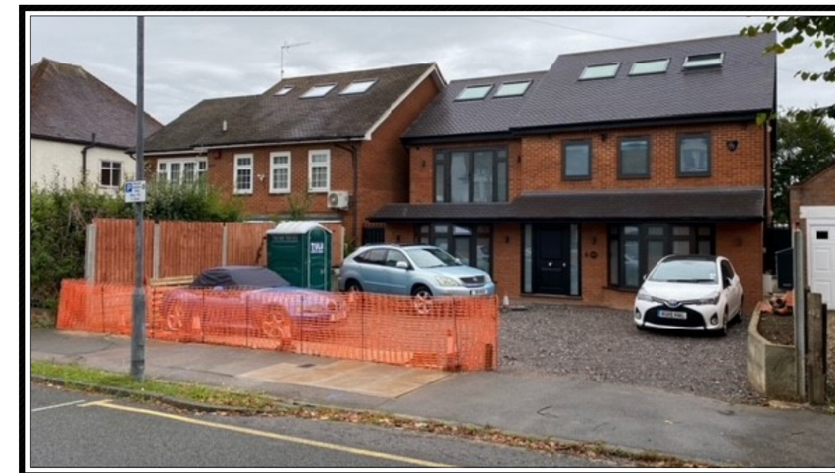
EXISTING STREET SCENE PHOTO
