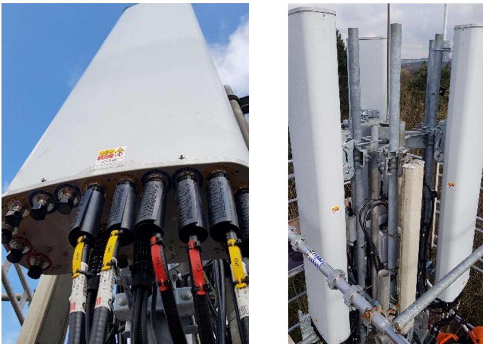
Source: Cellnex Trowell Services – 5G antenna and feeders
