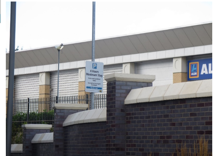
Reverse of wall above – facing pedestrians leaving car park to enter scheme
