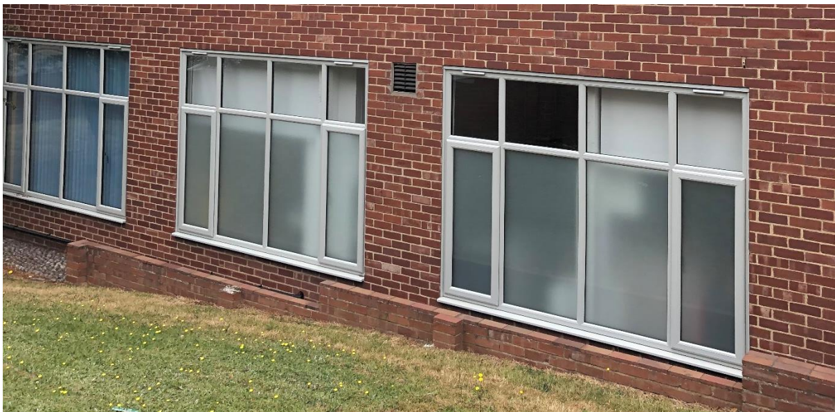
Figure 5: Proposed windows (already installed)
