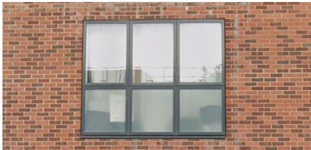
Figure 6: Grey windows at adjacent flatted development
