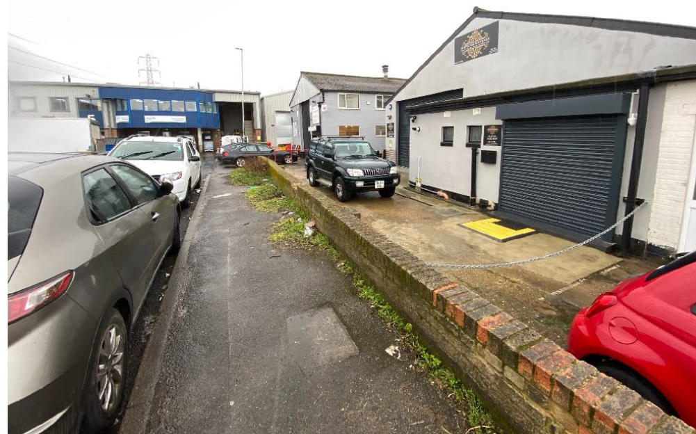
4. View looking south-east from the pavement towards the boundary wall, showing the level change across the driveway.
