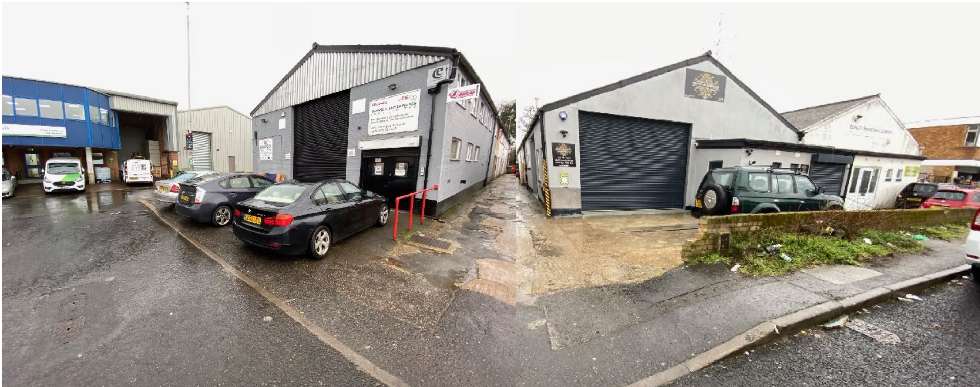
1. Panoramic view looking south-west Eskdale Road towards the front of application property No. 3a and neighbouring unit, showing the existing dropped kerb access.
