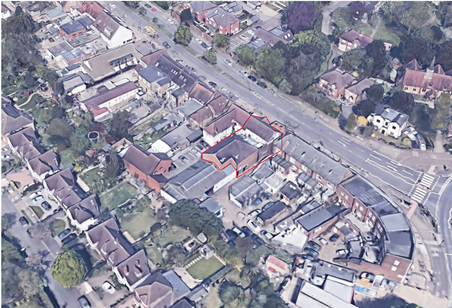
Existing aerial view from the South
