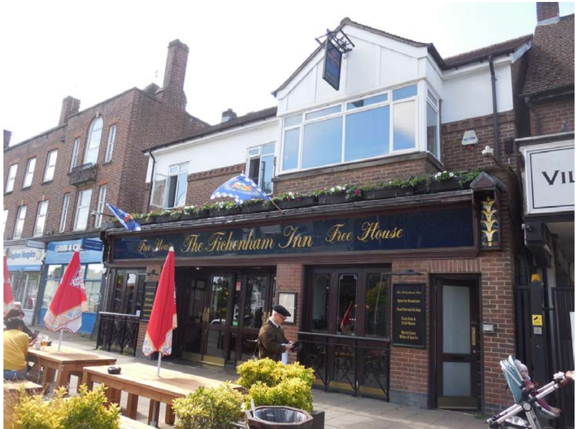
Front Street Elevation showing entrance to first floor flat.
