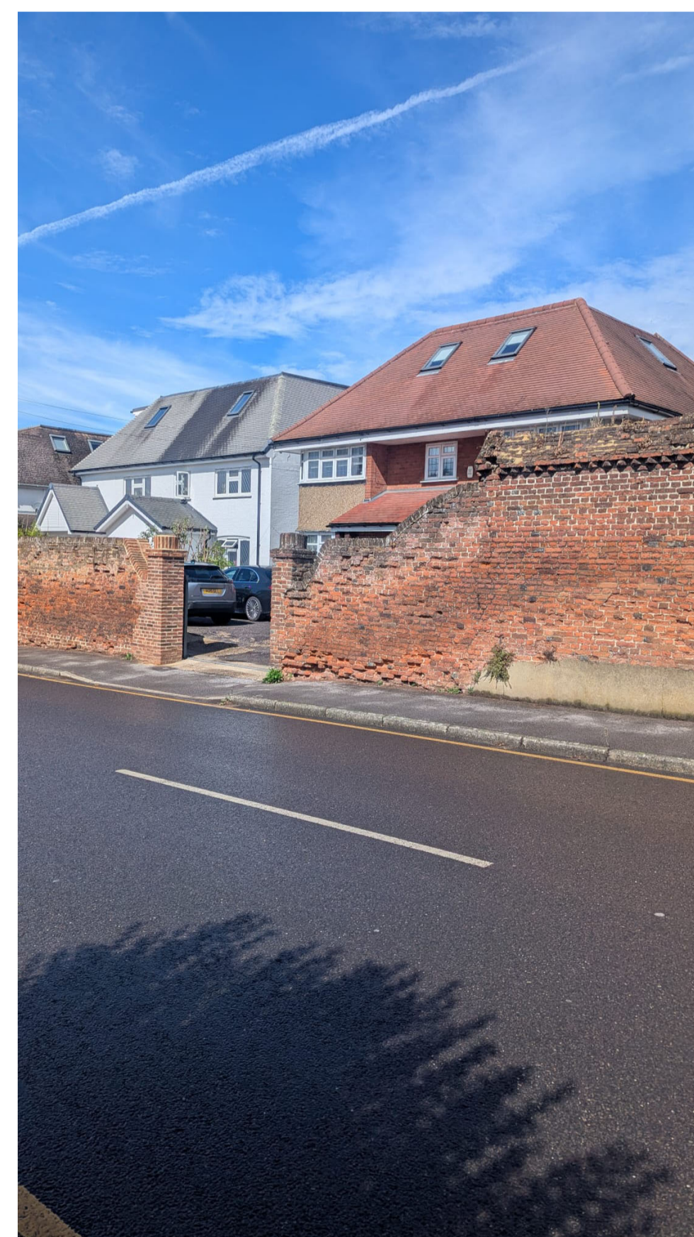
PHOTO 1: CHURCH RD VIEW TOWARDS NO. 28 AND NO.30
