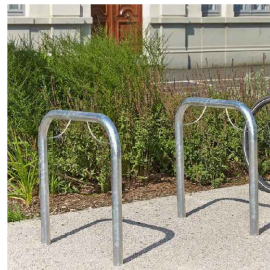
Sheffield cycle stand in stainless steel, from Broxap street furniture or similar and approved.
