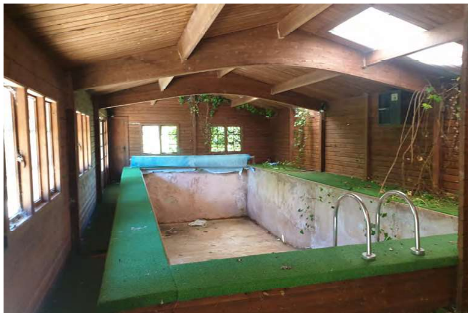
Pool building internals
