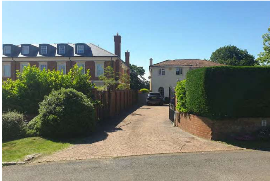
Front of the site and entrance looking west
