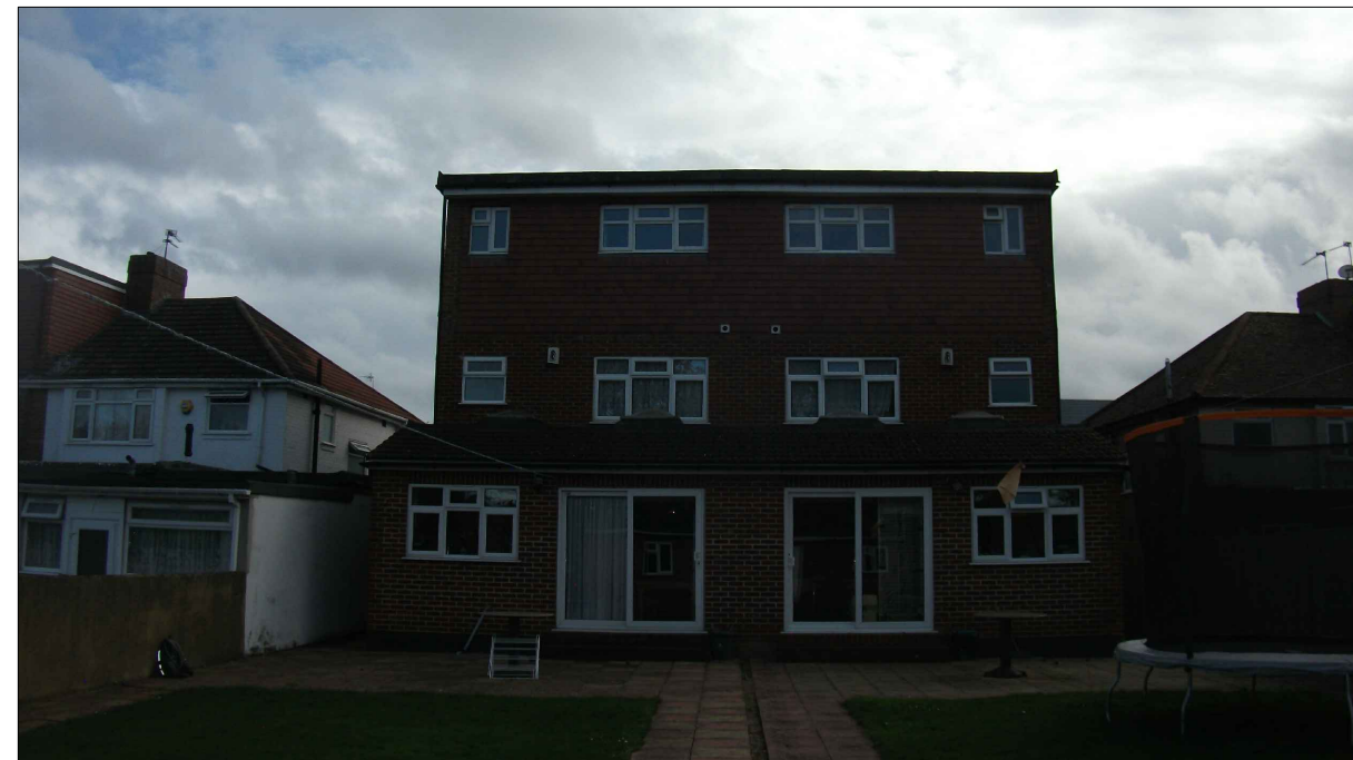
EXISTING REAR PICTURE
