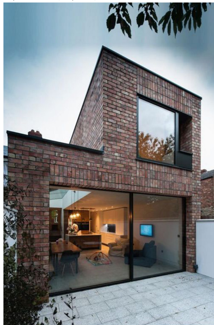
Smart Architectural Aluminium (or equivalent) brown-grey or black-grey aluminium door and window frames
