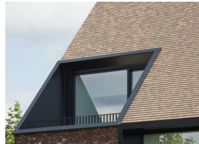
Marley Acme Double Camber Clay Plain Roof Tiles or equivalent concrete roof tiles
