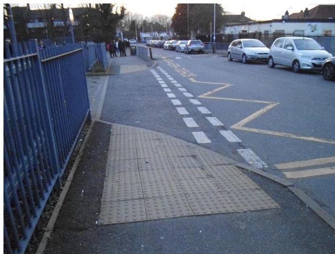
Photo 1: Pedestrian Infrastructure on Sidmouth Drive
