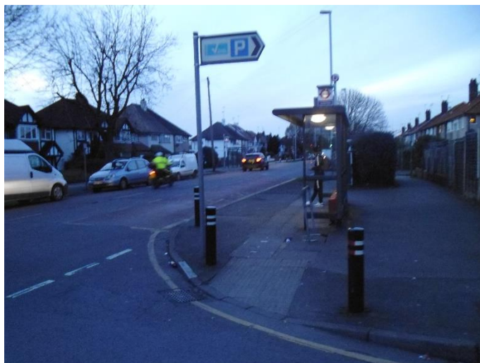
Photo 5: A1480 (West End Road) Bus Stop (Southbound)
