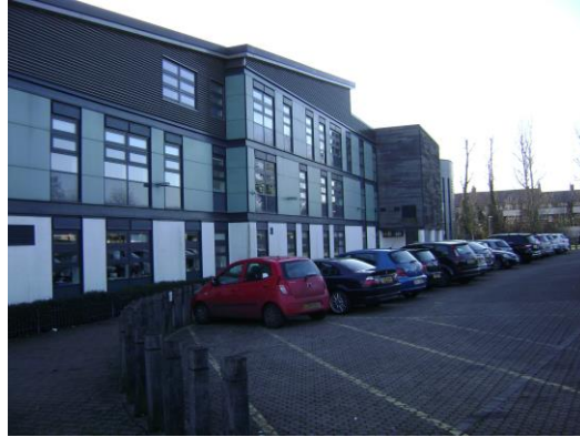
Photograph 2. Building on site
