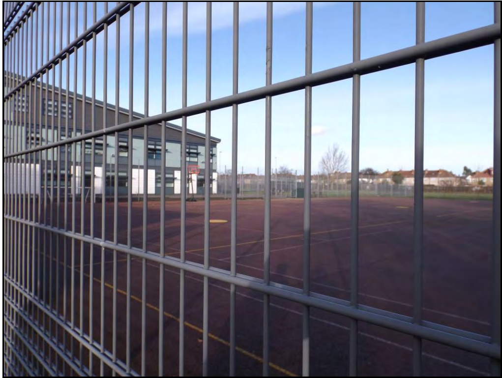
Plate 6: Rear all weather playing surfaces viewed from back of school buildings, looking northeast.
