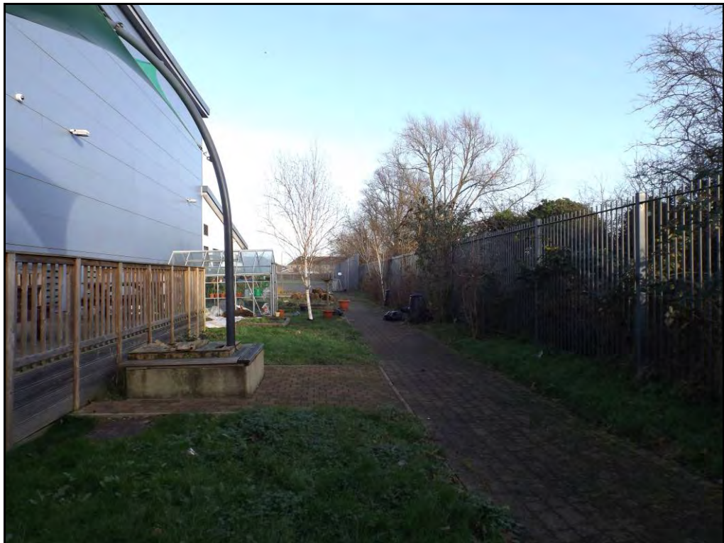
Plate 5: Southern/rear of school building, with decking and eco-area, looking east.
