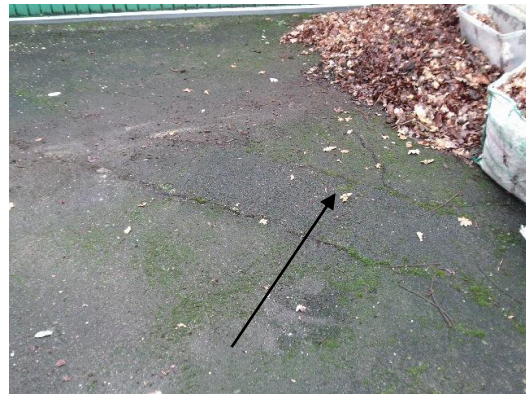
View of movement to tarmac driveway
