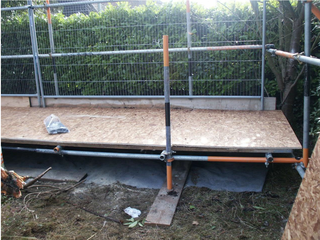
Photo 2 Scaffold framework supporting wooden boards
