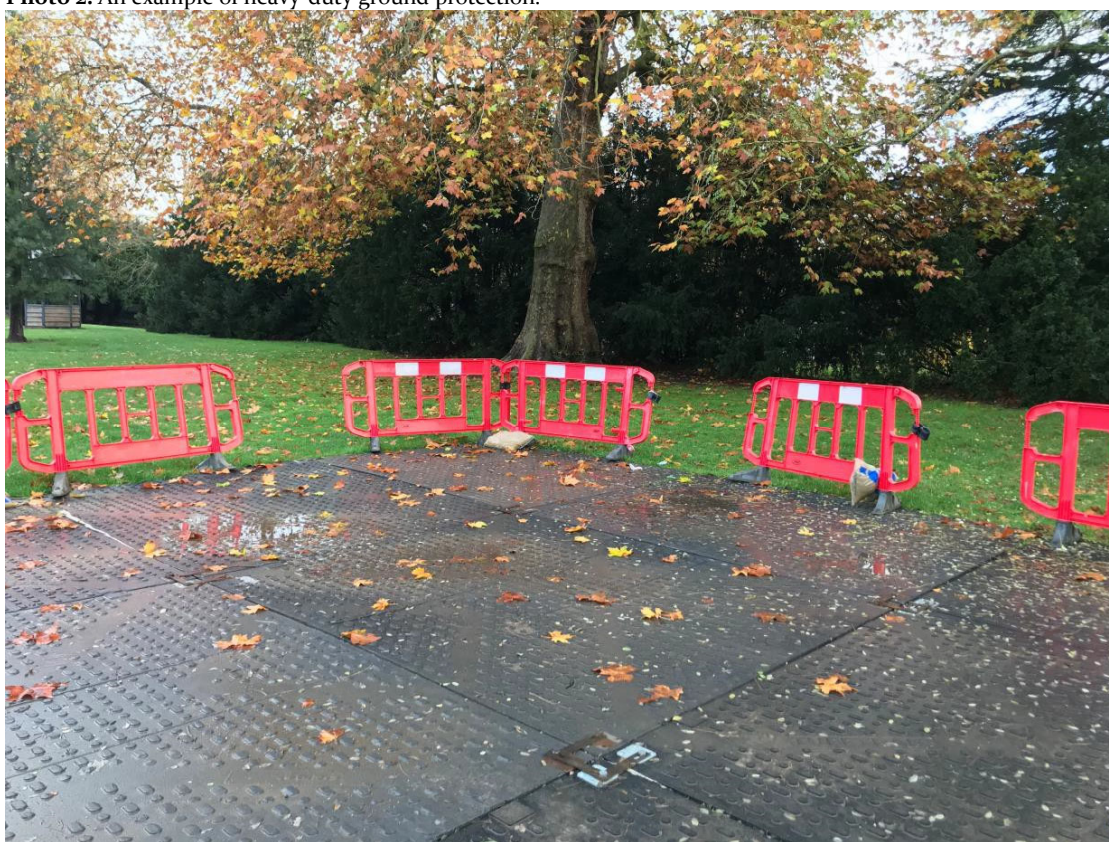
Photo 2. An example of heavy-duty ground protection.
