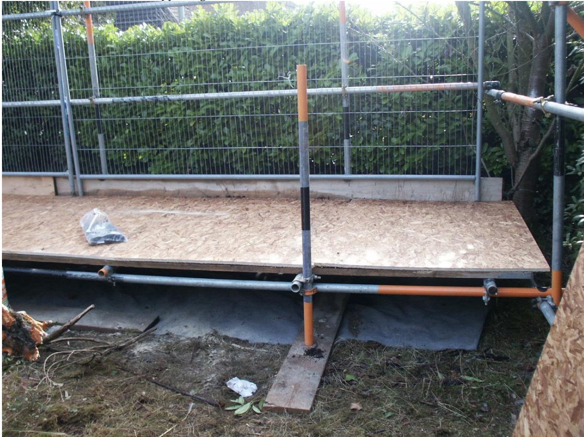
Photo 2 Scaffold framework supporting wooden boards
