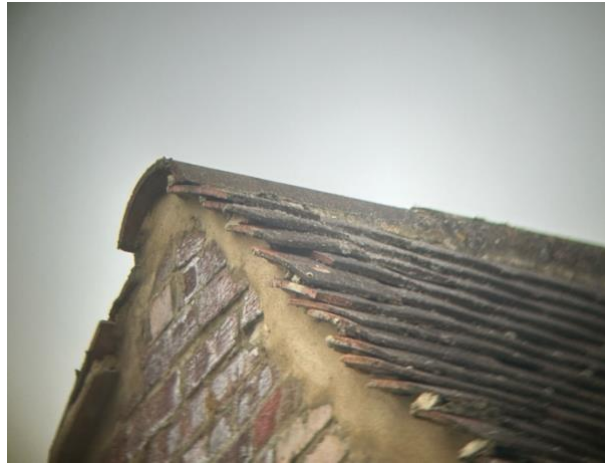
Figure 8. B1 – Lifted/dislodged roof tiles
