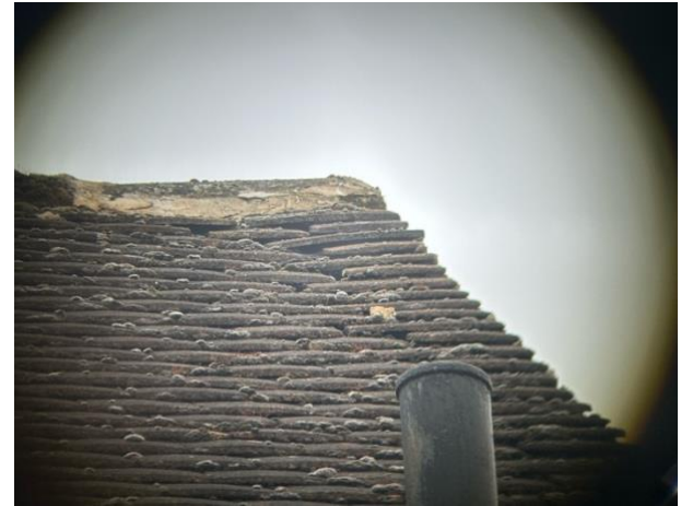
Figure 9. B1 – Lifted/dislodged roof tiles
