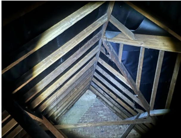
Figure 13. B1 – Loft space
