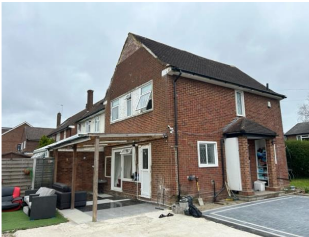
Figure 4. Facing northwest at B1
