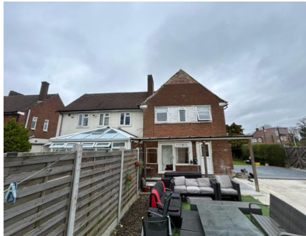
Figure 2. Facing north at B1
