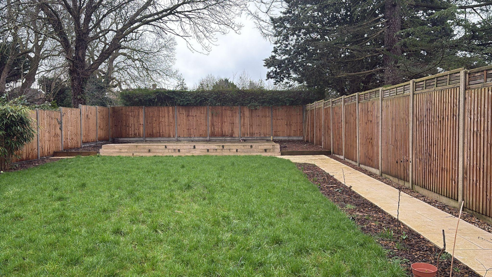
EXISTING BASE AT BOTTOM OF GARDEN WHERE GARDEN STUDIO IS PROPOSED
