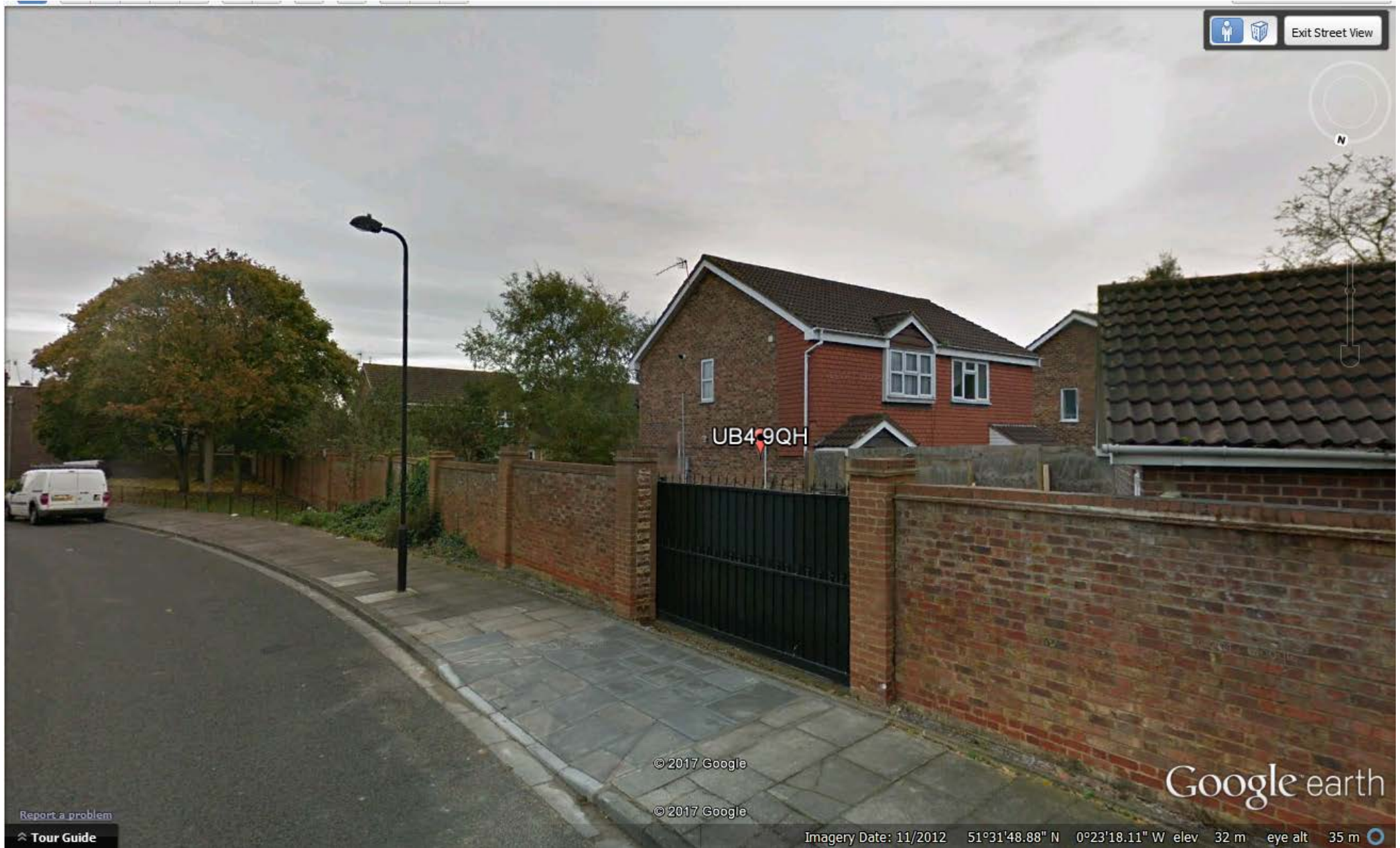
Figure 3 -Detail view - crossover to gates, boundary wall and flank wall/front elevation to No. 50/52.
