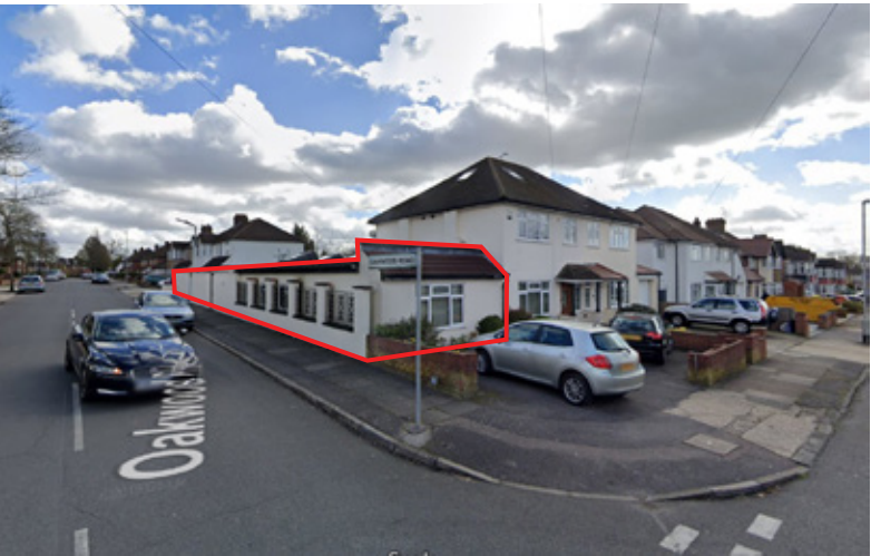
(above) Side extension to 9 Hazelwood Drive viewed from the front
