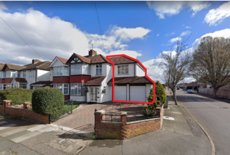
(above) Side extension to 31 Hazelwood Drive viewed from the front
