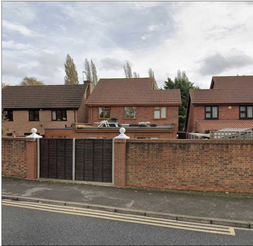
Figure 2: Image of the appeal site, viewed from Broadmead Road
