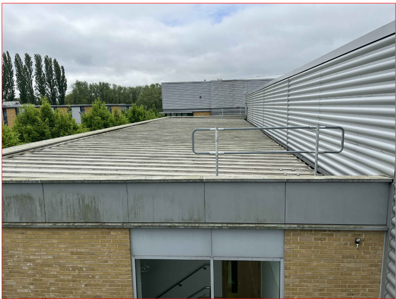
VIEW ON OFFICES ROOF
