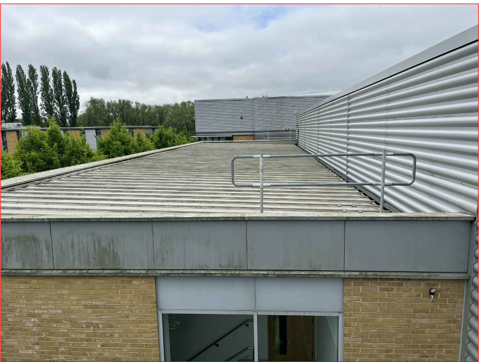
VIEW ON OFFICES ROOF
