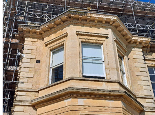
Image 8: Existing cornice to be replaced, windows to be repaired and glass to be replaced
