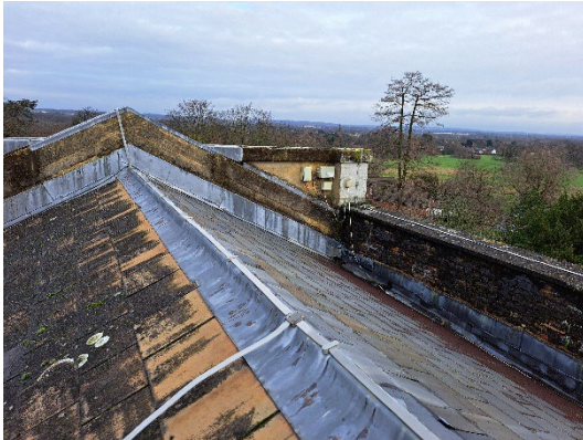
Image 1: Existing roof coverings to be replaced
