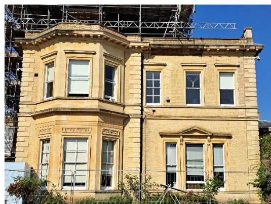
Image 12: Existing windows to be repaired and glass to be replaced
