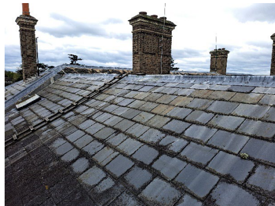
Image 4: Existing roof coverings to be replaced
