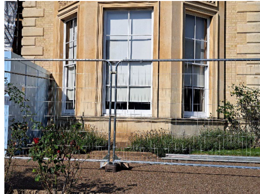
Image 10: Existing windows to be repaired and glass to be replaced
