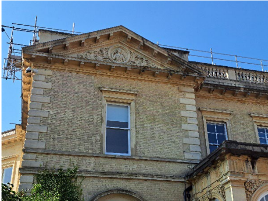
Image 13: Existing windows to be repaired and glass to be replaced; cornice to be replaced but original tympanum will be retained and conserved
