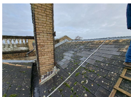
Image 6: Existing roof coverings to be replaced and chimney to be repaired
