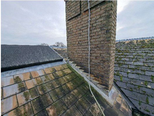
Image 7: Existing roof coverings to be replaced and chimney to be repaired
