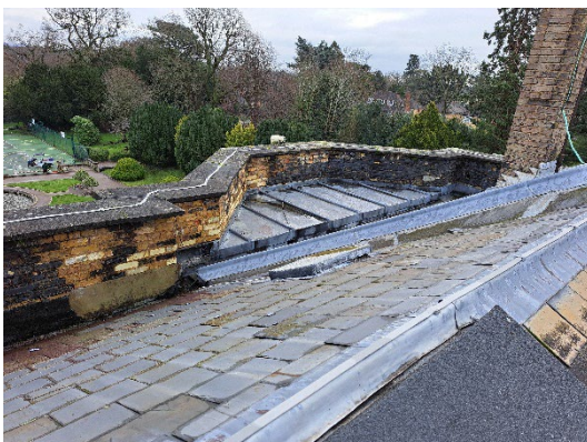
Image 5: Existing roof coverings to be replaced and parapet wall to be dismantled
