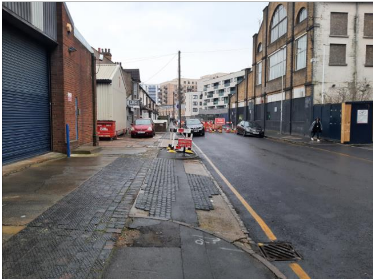
Photograph 5.2: Poor Surface Materials on Blyth Road
