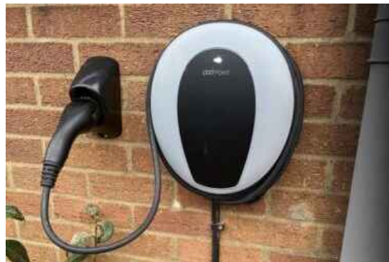
EVC charger from Pod Point Electric Vehicle Charger Tethered Solo 3 7kW wall mounted
