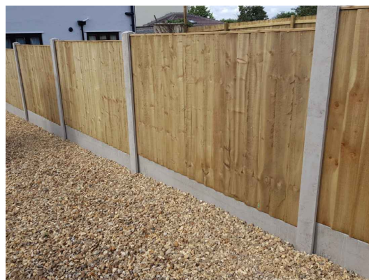
Timber fence Close boarded 1.8m timber fence with concrete posts
