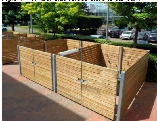
Fig.3.1 – Timber-clad refuse store to car park
