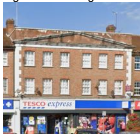
Fig.2.5 – building elevation to Field End Road shops in-front of the site.
