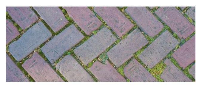
permeable paving to car parking/shared surface areas, entrance and ground floor terraces
