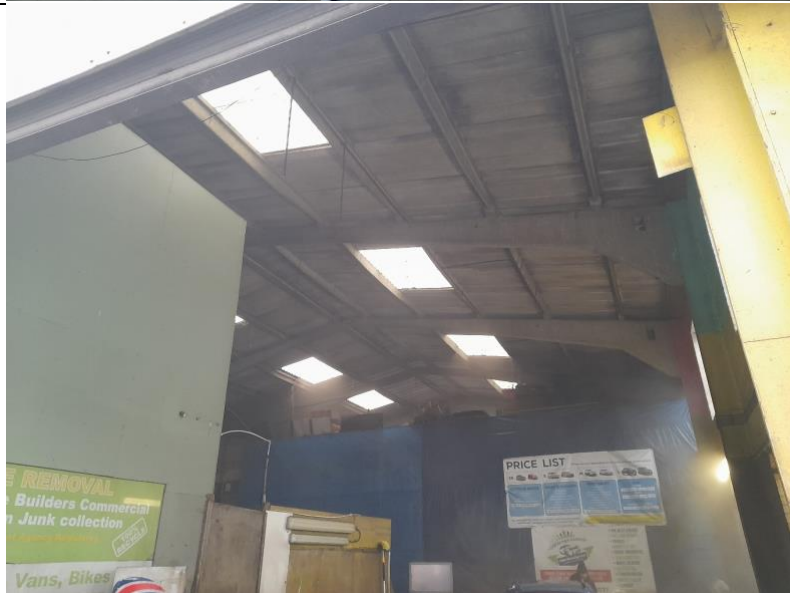
Photograph 2: Internal roof structure.
