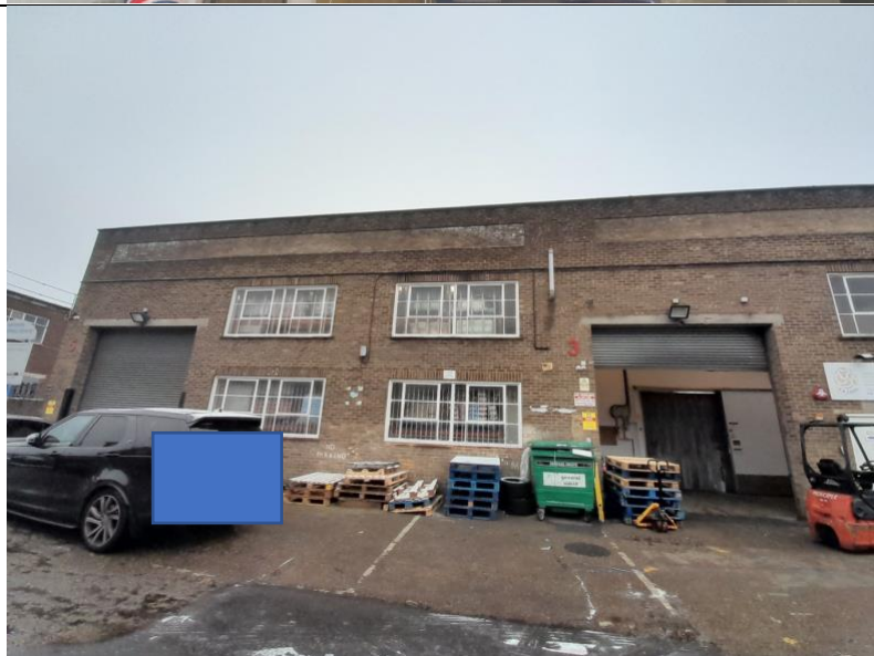
Photograph 3: External building structure
