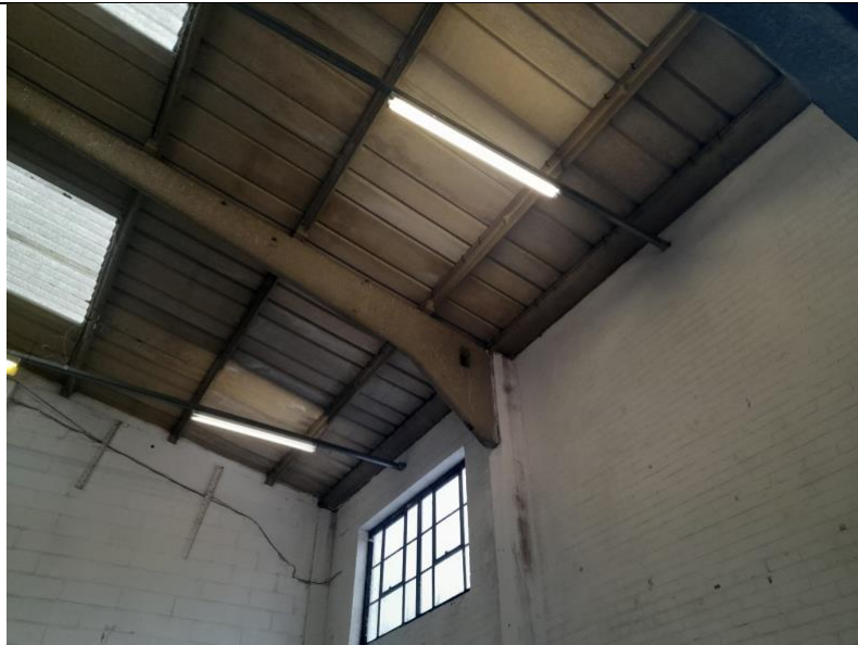
Photograph 1: Internal roof structure.
